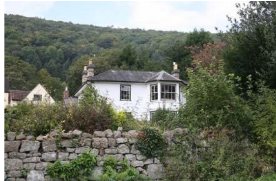
Fig.58 Dry stone boundary walls are important features throughout the Conservation Area
