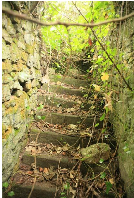
Fig.59 Footpaths are often enclosed to one or both sides by dry stone boundary walls and include important features such as stone steps
